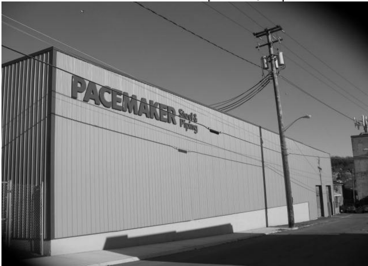
Pacemaker Steel & Piping Company Binghamton Plant
